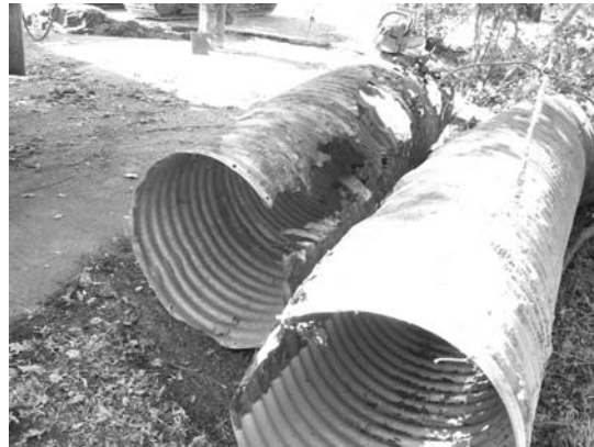
Rusted culvert removed from Mountain Pine
