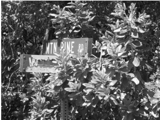
Deteriorated and obscured road sign
