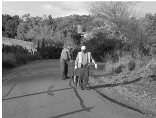
Javier and Hector seal cracks on Cedar Lane
