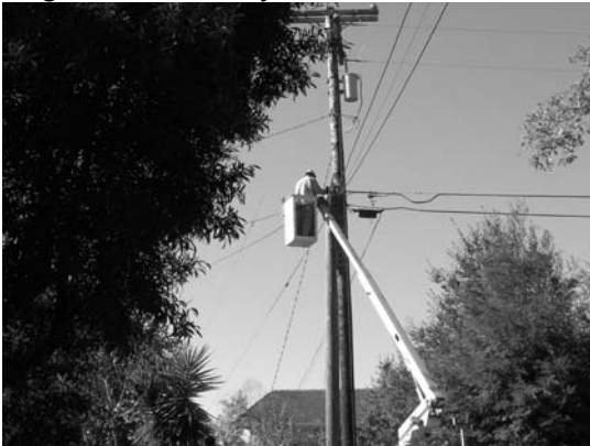
Comcast removes pole on Mountain Pine Rd
