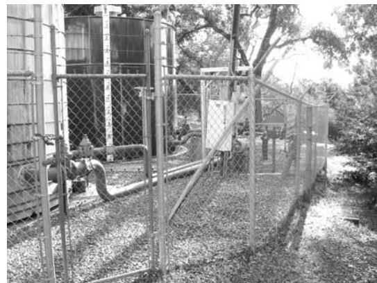
Tank#1 after clean up
