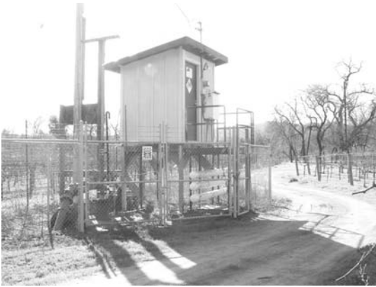
Existing well with proposed site in background
