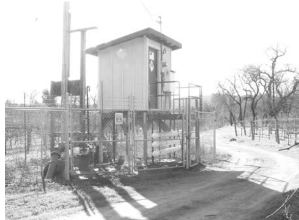
The Palomino Lakes well facility
